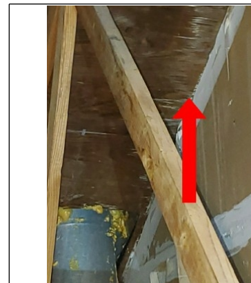
Inside damage noted from prior leak
