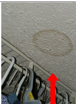
Following the leak, areas below moisture penetration in attic
