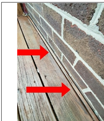
Ledger board not sealed / caulked / flashed to prevent moisture penetration.
