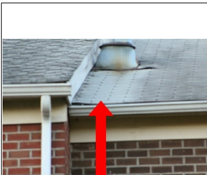
Evidence of prior leak and repair.
