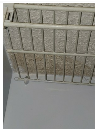
Inside damage noted from prior leak
